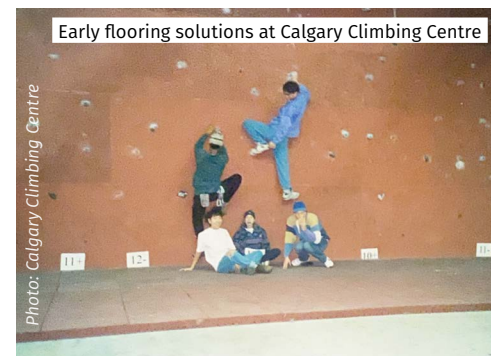
Crumb rubber floor with Cordless drag mats filled with scrap foam
